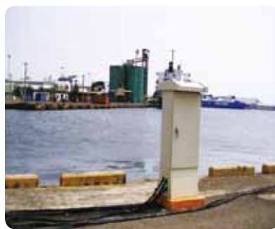
Shore power facilities, Port of Anping
