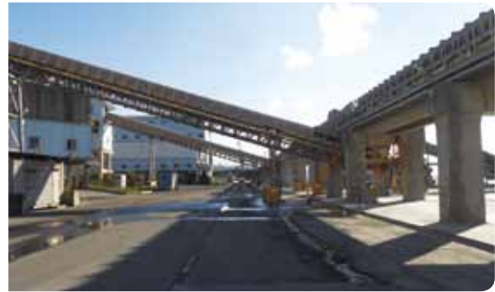
Berth E14 and E16 at the Bulk & General Cargo Terminal No.1 of Taipei Port has automated spiral coal and gravel unloader and conveyor system to mitigate dust concerns.
