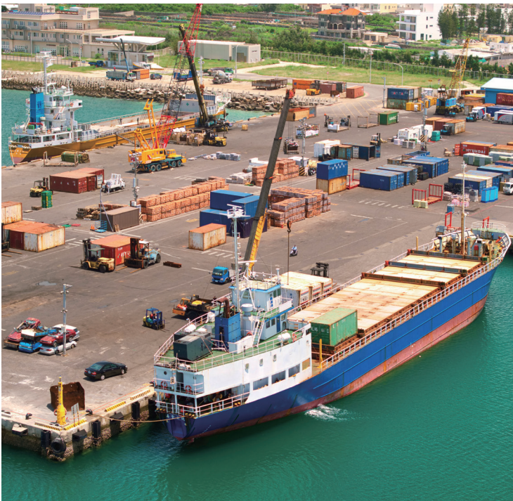
Longmen Jianshan Terminal Zone (Bulk Cargo Operation Wharf)
