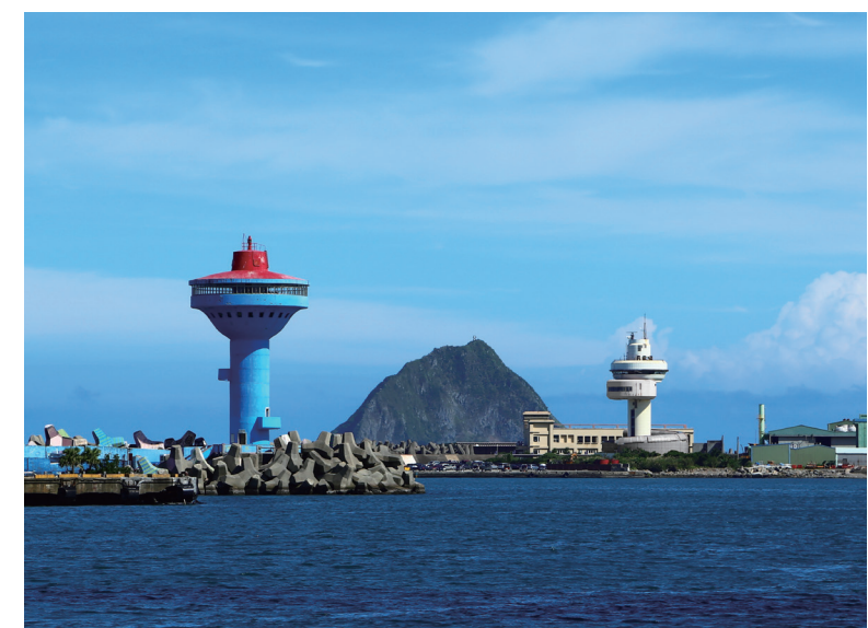
Harbor Guardian: Guan-Hwa Tower & Vessel Traffic Service
