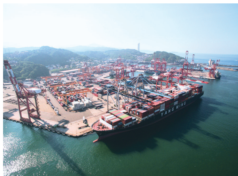
West Coast Container Terminal
