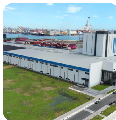
Kaohsiung Port's A6-A Submarine Cable Base Supports Taiwan's Green Energy Transition
