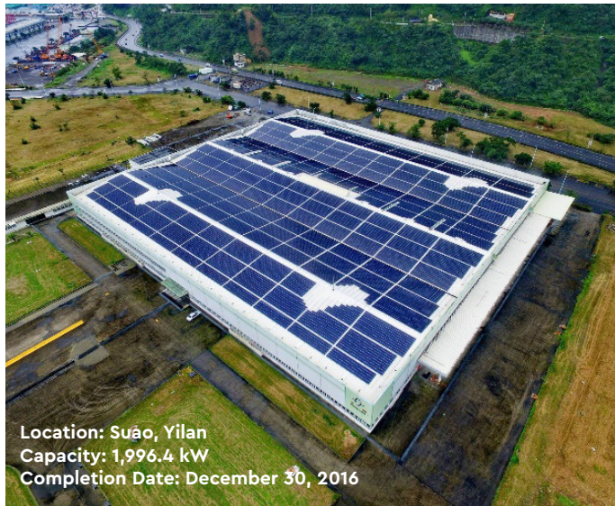
Photovoltaic System on the Roof of Pihsiang Machinery
