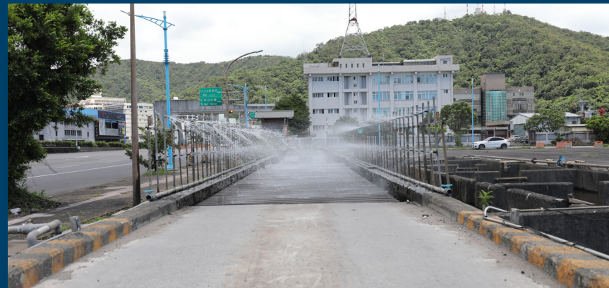
Sensor-activated vehicle washing station (utilizing recycled spring water)
