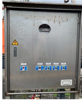
Shore Power Facilities at the Barge Wharf
