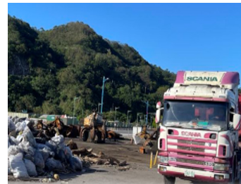
Removal of large volumes of waste generated by typhoons
