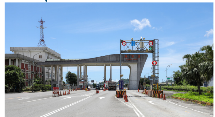
Inbound trucks are inspected through the Automatic Gate Sentry System.
