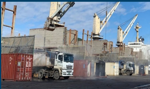
Install dust screens at cargo handling piers for fugitive particulate materials
