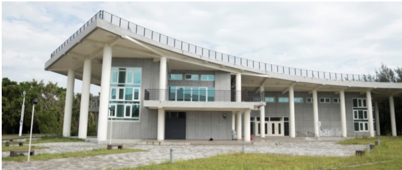
Green Building of Nanxing Management Center
